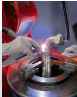
TIG welding capabilities according to the most demanding certifications
